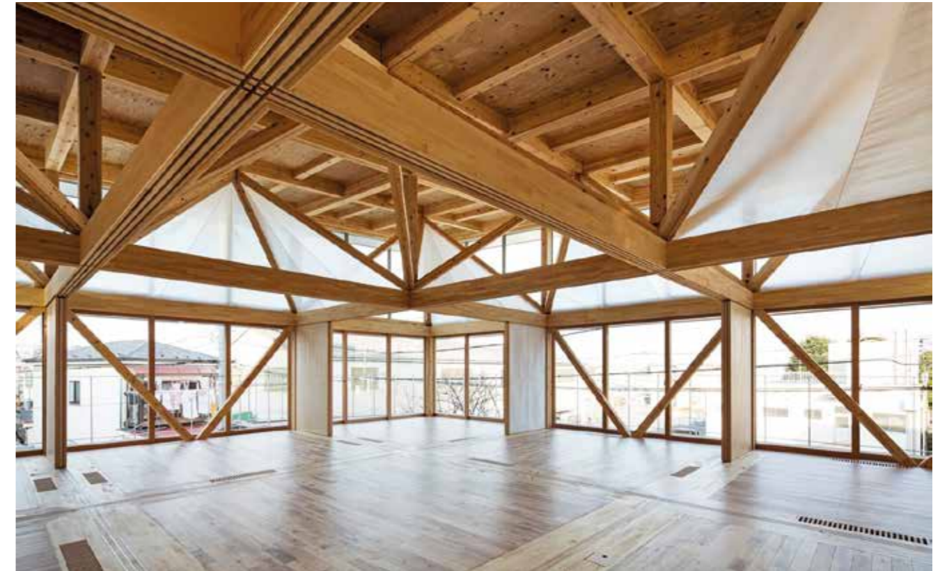
Abb. 12 Substrate Factory Blick ins Obergeschoss
